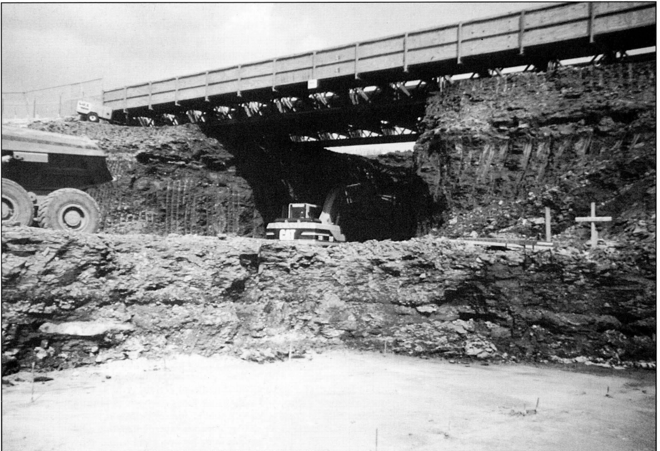
Fig. 2. Temporary overbridge of A607 road, supported on the Marlstone Rock Formation (upper strata) overlying Brant Mudstone Formation. The concreted foundation for the permanent bridge is in the foreground.
